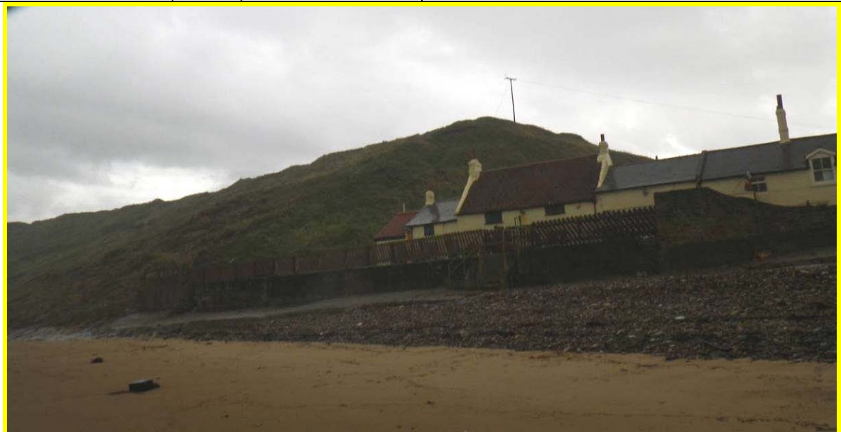
E53/5 has slumped, leaving open cracks in the cliff face and resulting in instability classified as Locally Active.
