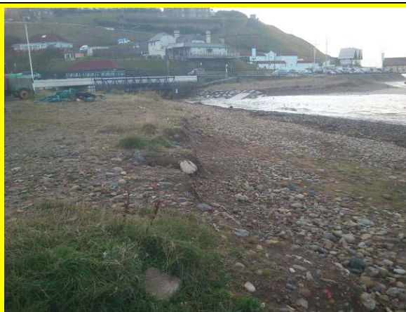
Evidence of previous storm damage to shingle bank at boat park (Asset Ref No 1221C901C0704C02)
