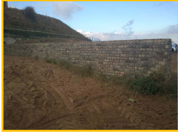
Wall enclosing fishing boat park (Asset Ref No 12221C901C0702C02)
