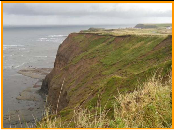
E59/4 fresh failures within the till and rockfall from lower cliff face (Partly Active)
