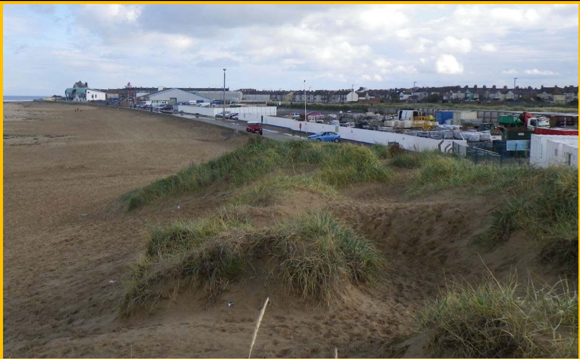
Overview of defences at west of Redcar from sand dunes adjacent to contractor's compound
