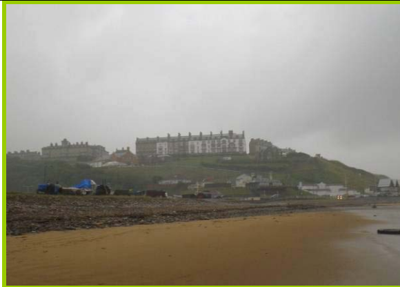
E52/2 the stable cliffs above Saltburn Sands (Inactive)
