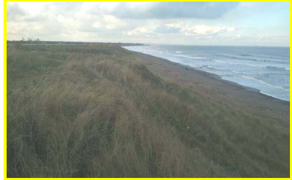
E52/9 Cobble beach gives some protection to Locally active cliff
