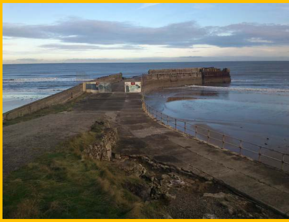
Jetty – view from south showing open gates (Asset Ref No. 1221D901D0201C02)
