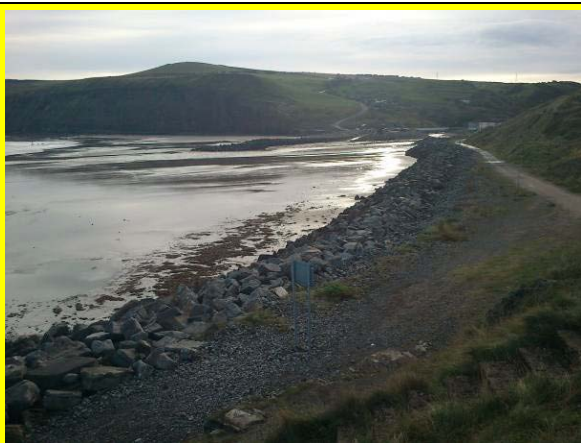
General view of rock armour revetment, from jetty to village (Asset Ref No. 1221D901D0202C01)
