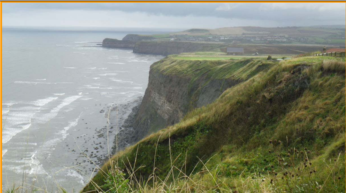
E59/8 looking towards Staithe from Boulby (Partly Active). Cowbar Nab in middle distance.
