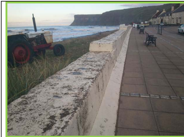
Set back rendered wall protected by shingle beach (Asset Ref No 1221C901C0704C03)
