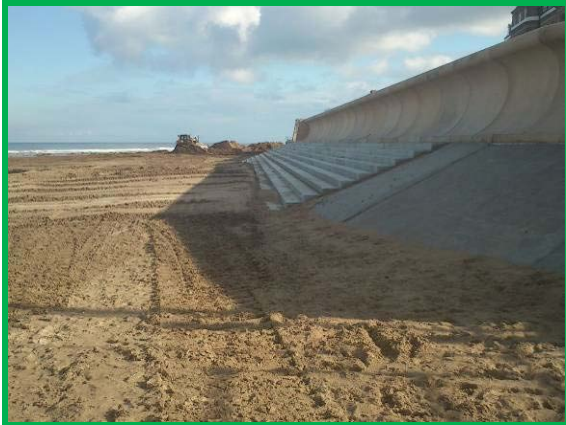
Works underway at west end of Redcar seawall, Asset ref. 1221C901C0602C06
