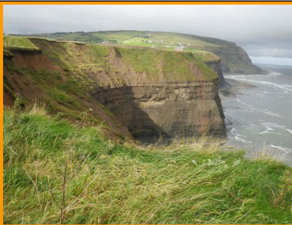
E59/5 failure and active headscarp recession within the upper till part of the cliff (Partly Active)
