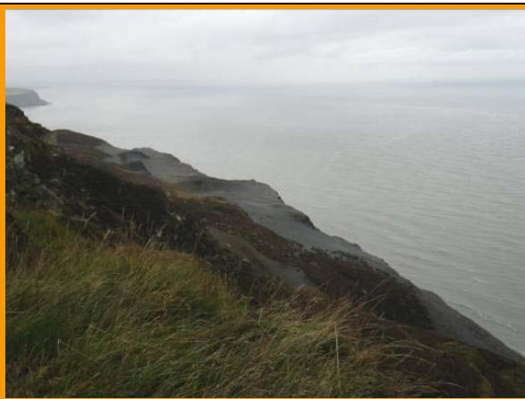
E58/5 Lower, is not vegetated and is prone to wave attack at the toe.
