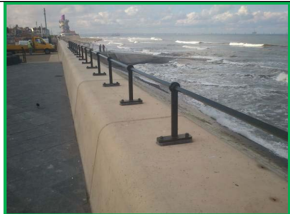
New crest wall adjacent to Esplanade, Asset ref No. 1221C901C0602C02
