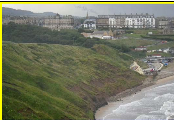
E53/4 Slumping in the till layer of the cliff northeast of Saltburn (Locally Active).
