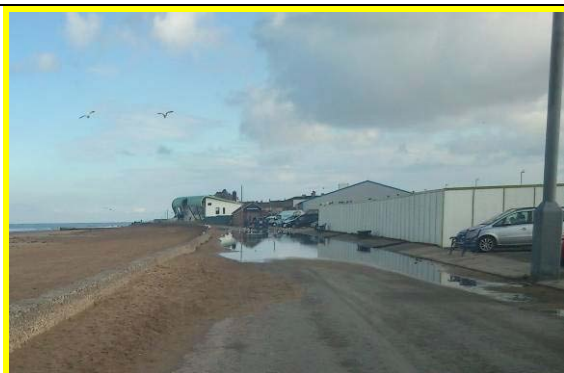
Flooded promenade due to blocked drainage (Asset Ref No 12221C901C0601C01)
