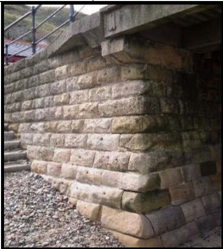
Photo from 2010 inspections
