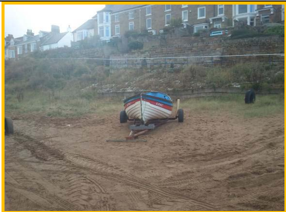
Extensive vegetation growth on revetment; local settlement of masonry structure similar to 2010. (Asset Ref No 12221C901C0702C02)
