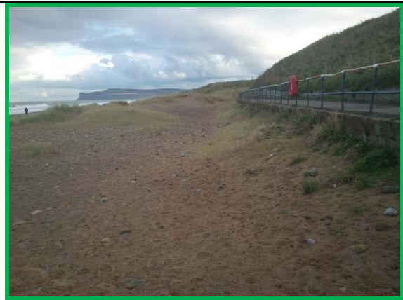
E52/7 Sand dunes and walls to toe of vegetated slope (Dormant) Photo October 2012
