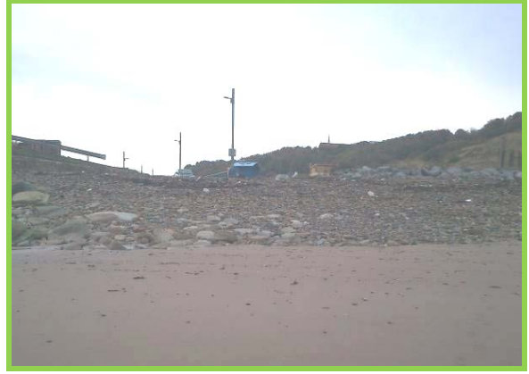
Shingle ridge looking landwards. (Asset Ref. No 1221D901D0202C04)
