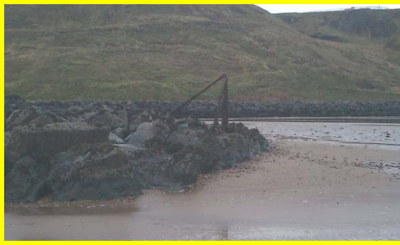
Seaward end of fishtail breakwater showing damaged navigation marker (Asset Ref No. 1221D901D0202C05)
