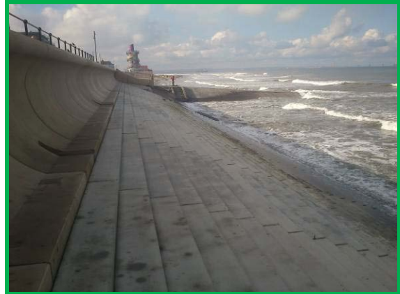
New stepped concrete seawall wall adjacent to Esplanade, Asset ref No. 1221C901C0602C02
