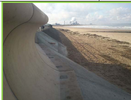
Interface with new seawall at the eastern end of Asset Ref No 12221C901C0601C01
