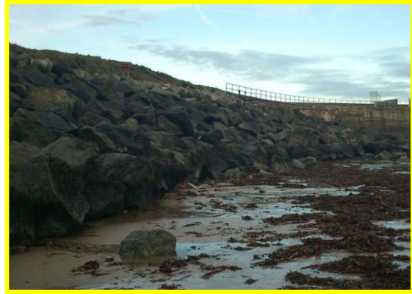
View of rock armour looking towards jetty (Asset Ref No. 1221D901D0202C01)
